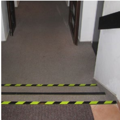
an obstacle in the form of uneven floor level hindering movement in wheelchair
